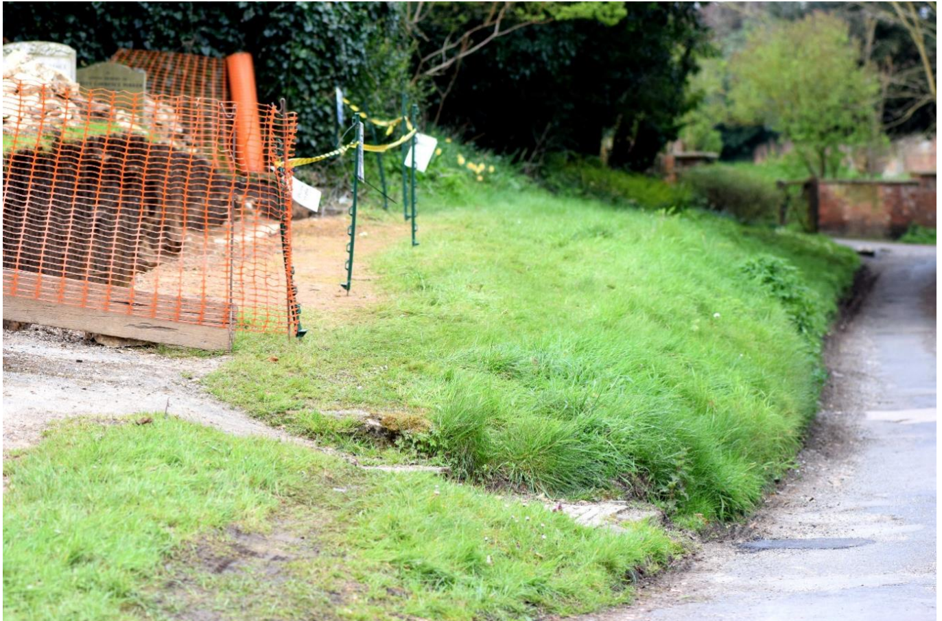
Fig 1. Boundary wall section at St Peter's Church boundary wall, Little Comberton, 21 April 2016, developed on a knoll of gravel soliflucted from the Pliensbachian of Bredon Hill's northern escarpment. Looking north-west the sediments have been incised at the edge of Manor Lane and changes in slope and altimetry are clear.
