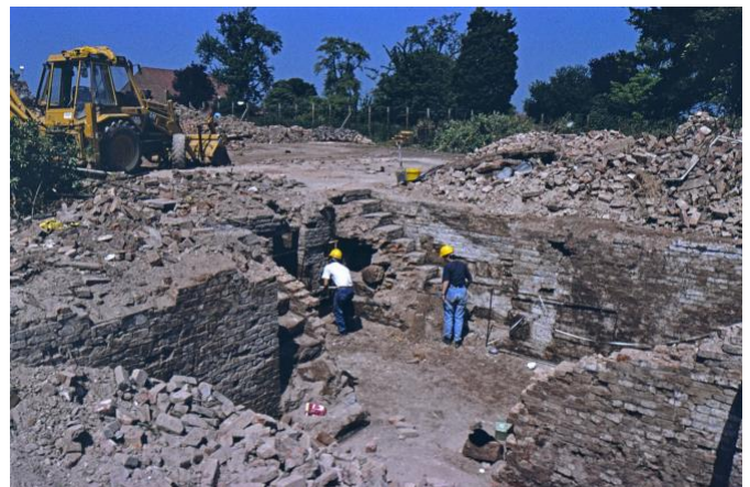
05. Lyppard Grange cellar excavation 1996. Will Watson.
