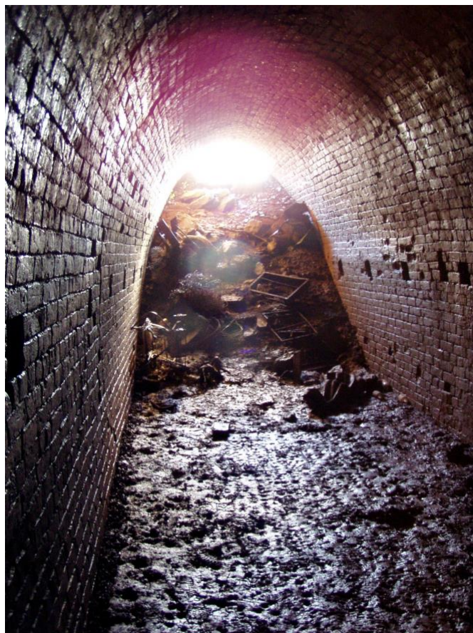
03. Inside Newnham Tunnel looking back to the entrance. Mike Averill.
