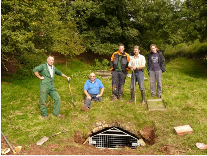
04. Newnham Tunnel after fitting Bat Grill 2008. Mike Averill.
