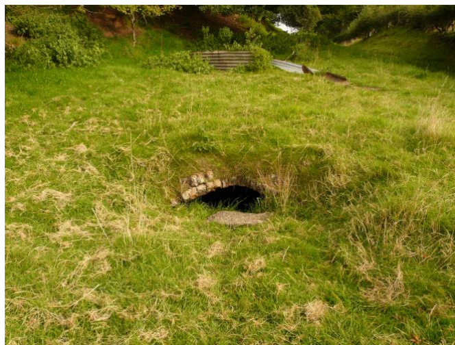
02. Newnham Tunnel entrance before fitting the grill 2008. Mike Averill.
